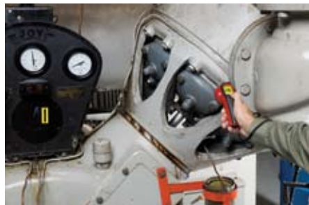
Diagnose temperature of wearing parts for preventive plant maintenance.
